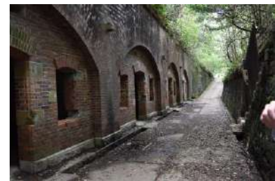
友ヶ島第3砲台
