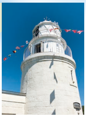
4 Tomogashima Islands Lighthouse: A chalk lighthouse that is still in operation today.
